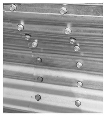
Install tarp hooks at bottom of circle. After every panel joint, install one panel hook; then leave 2 spaces between the remainder.
