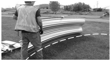
Once aligned, drive a strut into the ground (inside circle) and bolt it to 2 humps of panel.
