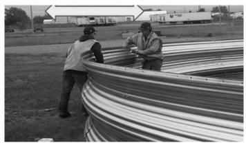
7. Once panel is aligned install strut (there should be a strut every second panel)
